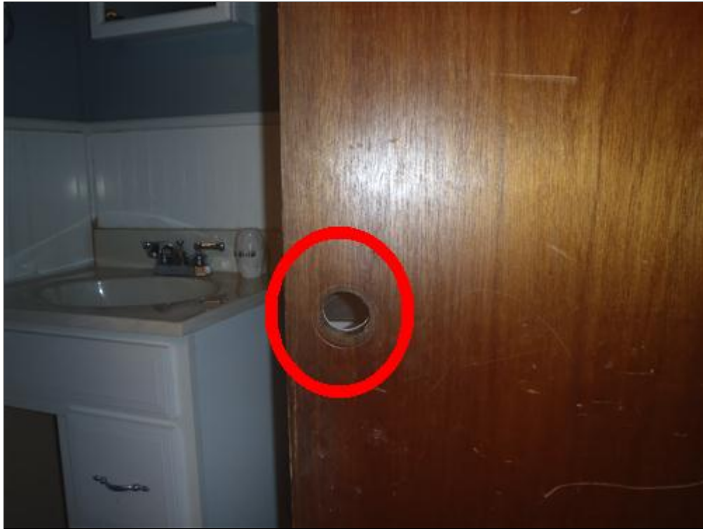
4.5 Picture 1 Basement door
