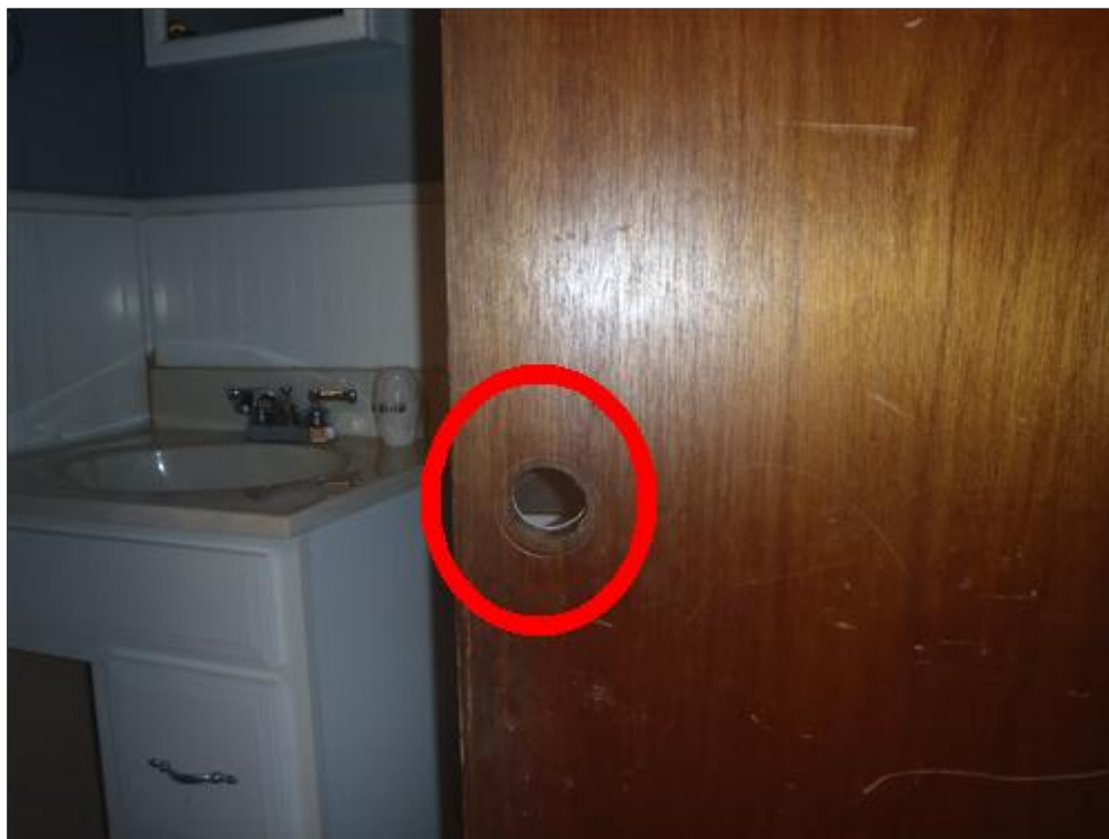
4.5 Picture 1 Basement door
