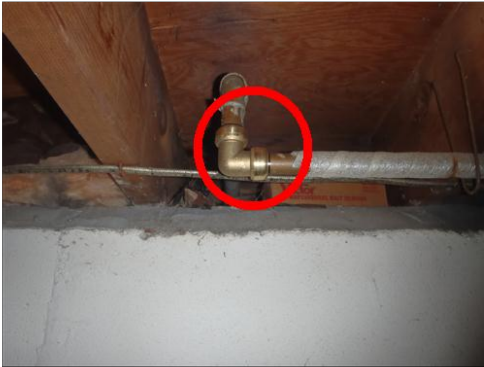
8.3 Picture 1 Shark bite repair
