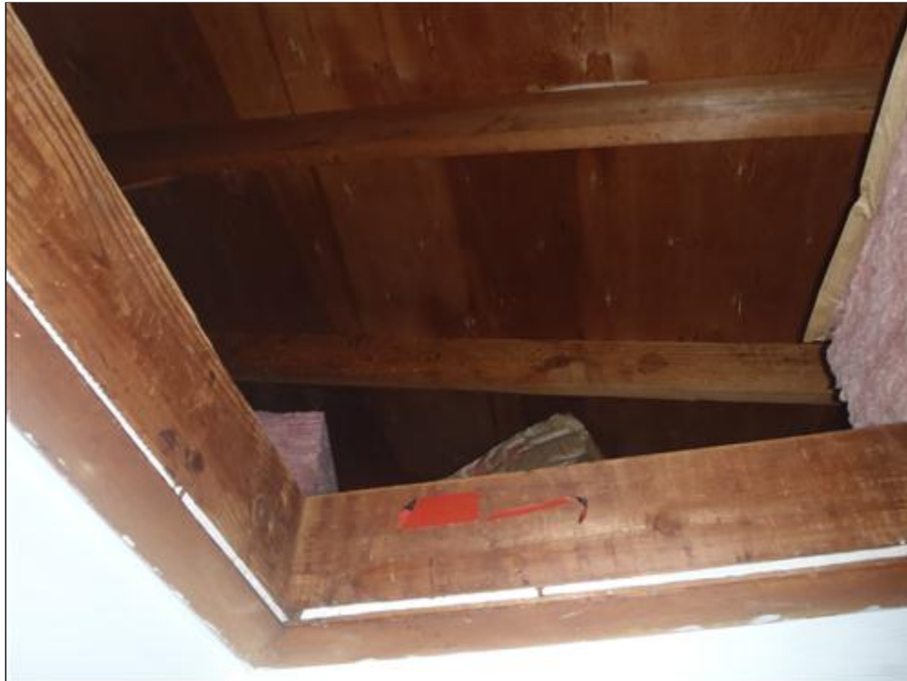
1.16 Picture 1 Attic hatch
