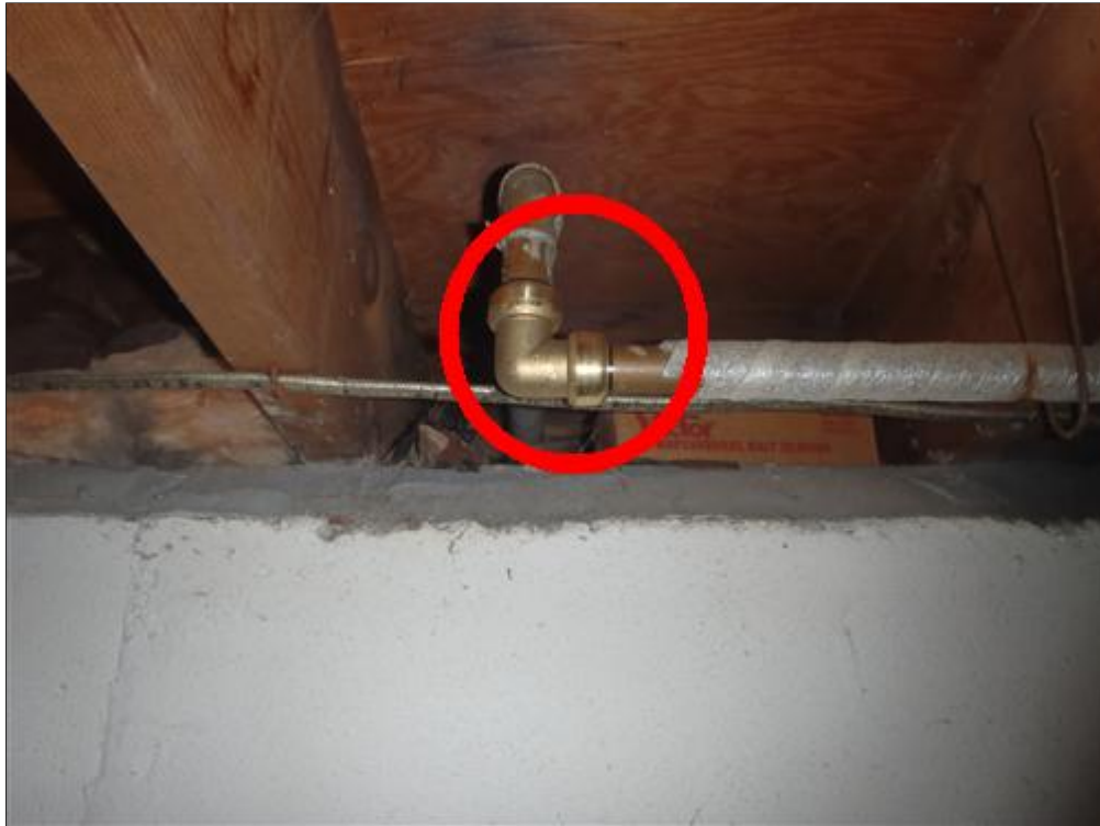
8.3 Picture 1 Shark bite repair
