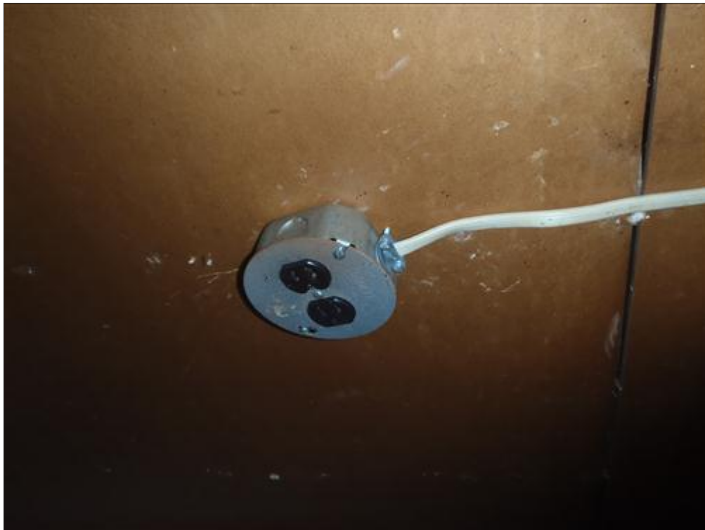
7.3 Picture 3 Garage ceiling
