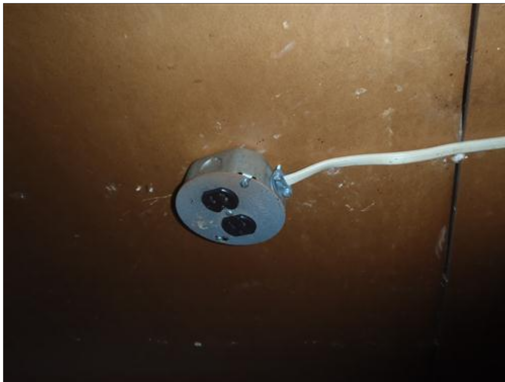
7.3 Picture 3 Garage ceiling
